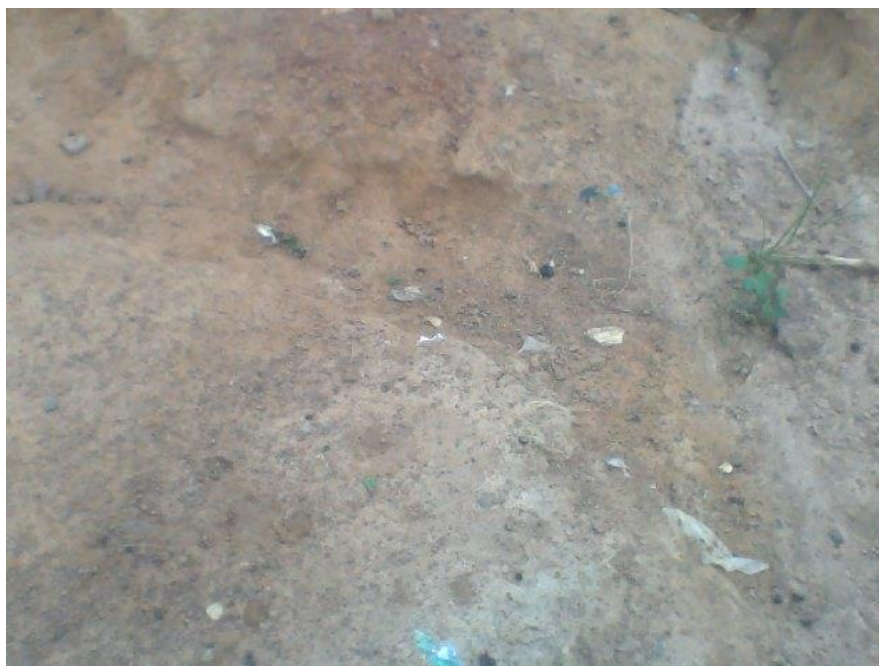
Erosion sides captured in Mayo-kam near Primary School
