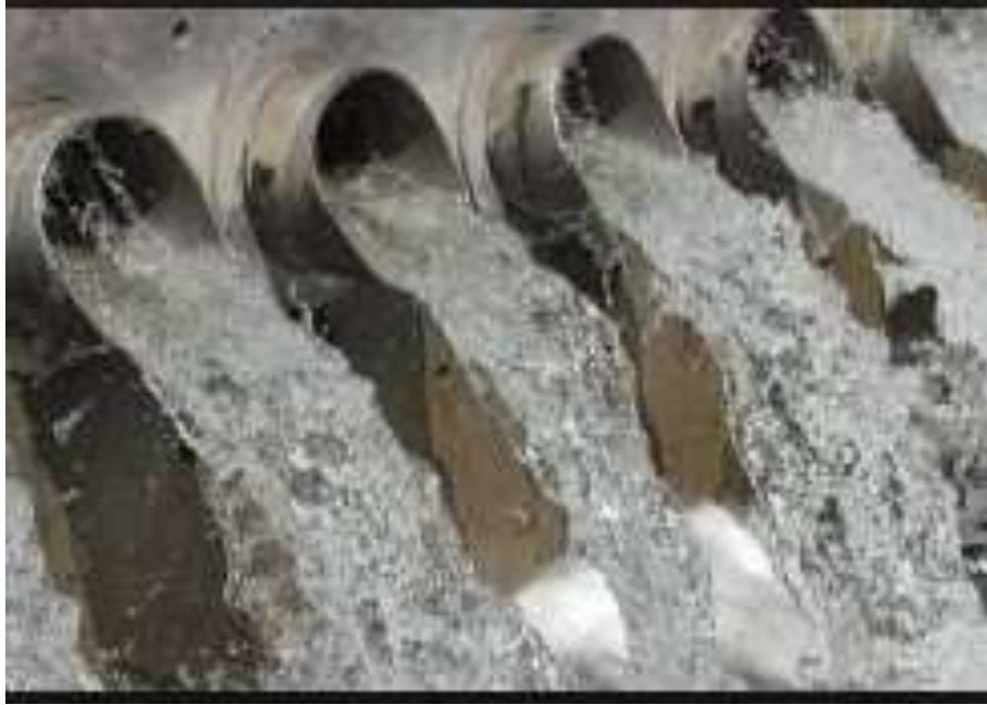
Figure 1: Waste water discharge weir
