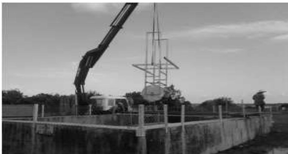
Figure 3: Installation of the system using a crane
