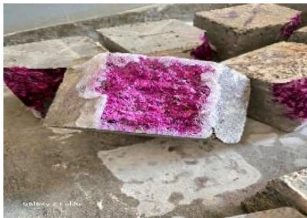
Plate 2: Showing a concrete cube showing reaction to carbonation depth.
