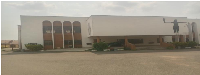
Plate 5: Exterior view of the Osun State High Courts of Justice
