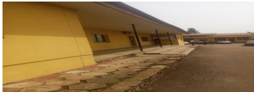
Plate 8: Entrance of the Ondo State High Courts of Justice
