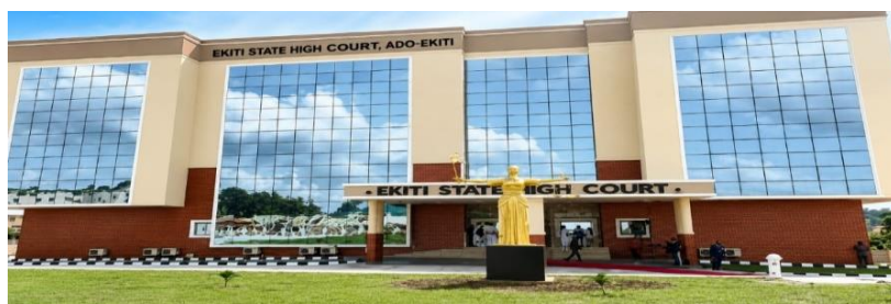
Plate 10: Approach View of the Ekiti State High Courts of Justice
