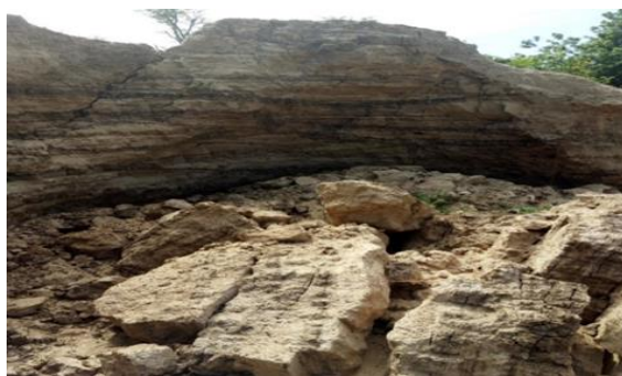
Figure 8: Land slide Caused by Mining of Pit Sand Source: Field Survey, 2026
