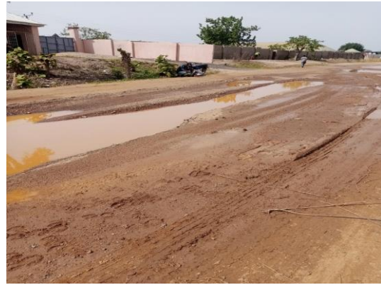
Plate II: Poor drainage
