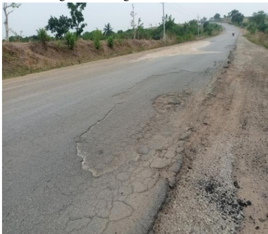
Plate III: Edge failure/deterioration
