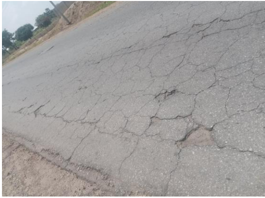
Plate I: Alligator cracking
