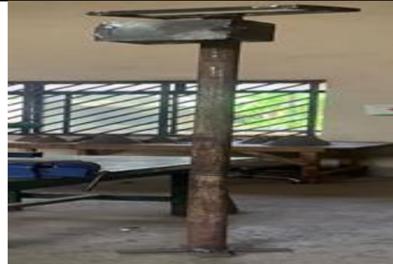
Figure 11: Automatic Solar Powered Streetlight Fabricated Pole
