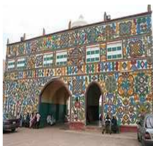
Plate 2: Emir of Zaria's Palace, showing traditional architectural wall finish.
