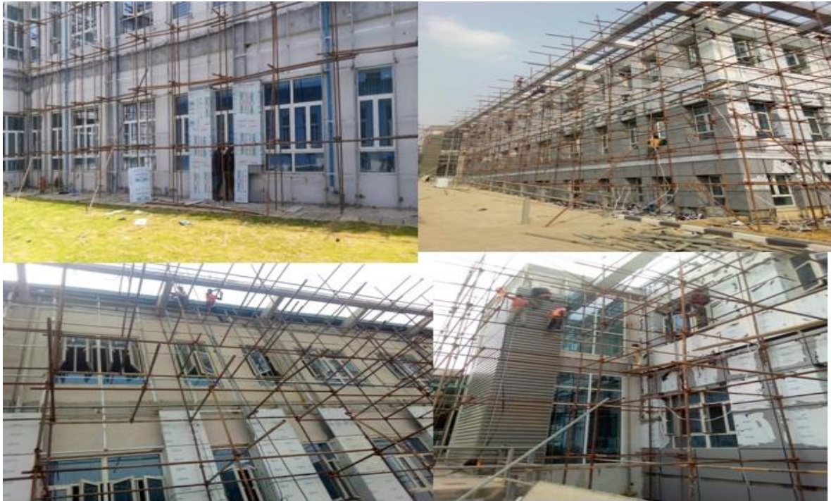
Figure 14: Cladding Activities at Various Stages
