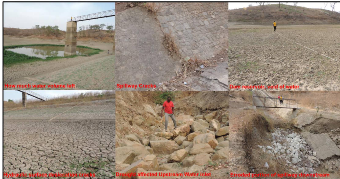
Plate 1: Different Aspects of Bosso dam Deficiency
