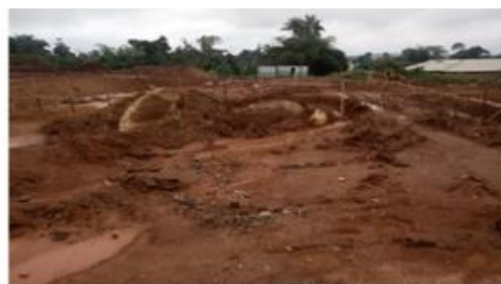
Figure 4c: Front view of proposed FL site
