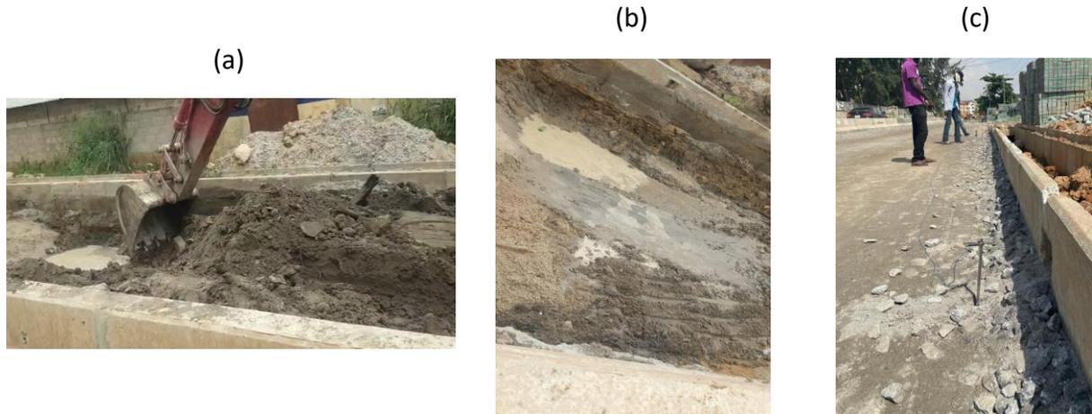
Figure 5: (a, b) Excavation of Clayey/Peat section along Traverse 1 during construction (c) A stable section of the road
