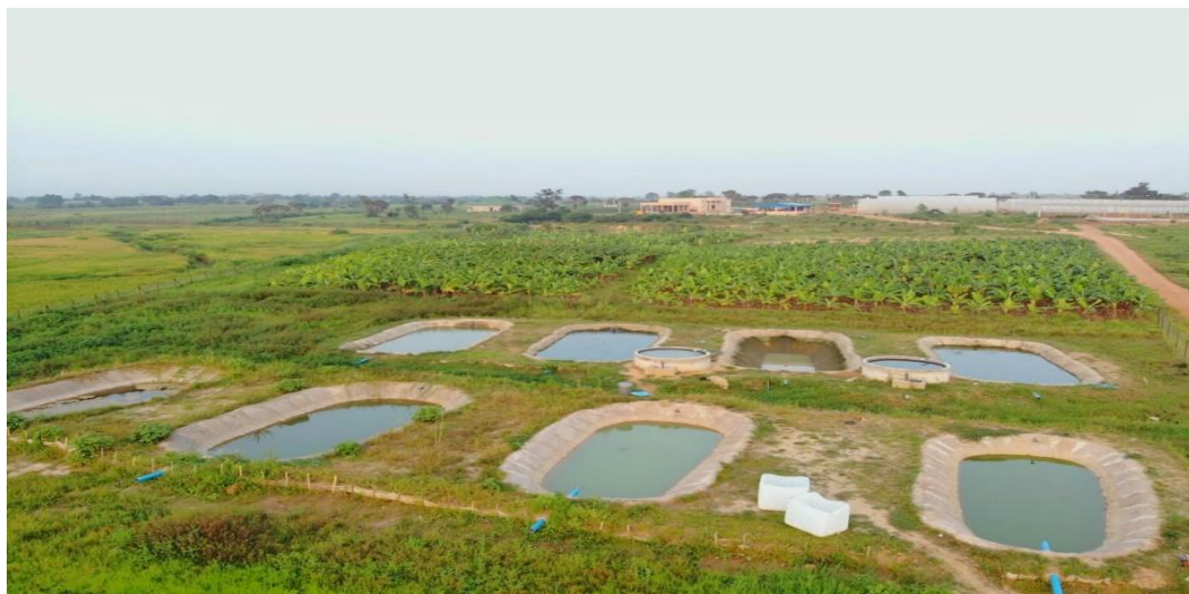
Figure 1: Aerial view of CDA Farm fish ponds
