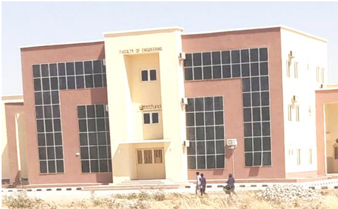
Plate 1: Faculty of Engineering Building, FUDMA
